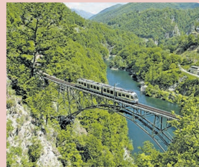
Centovalli Bahn Palagnedra
